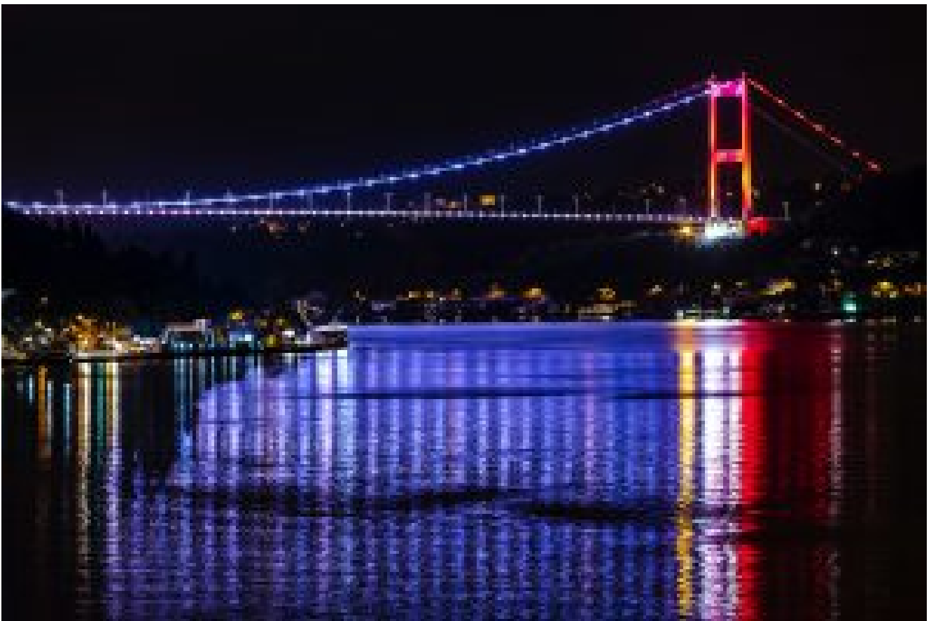
Bridge © Hulki Okan Tabak
