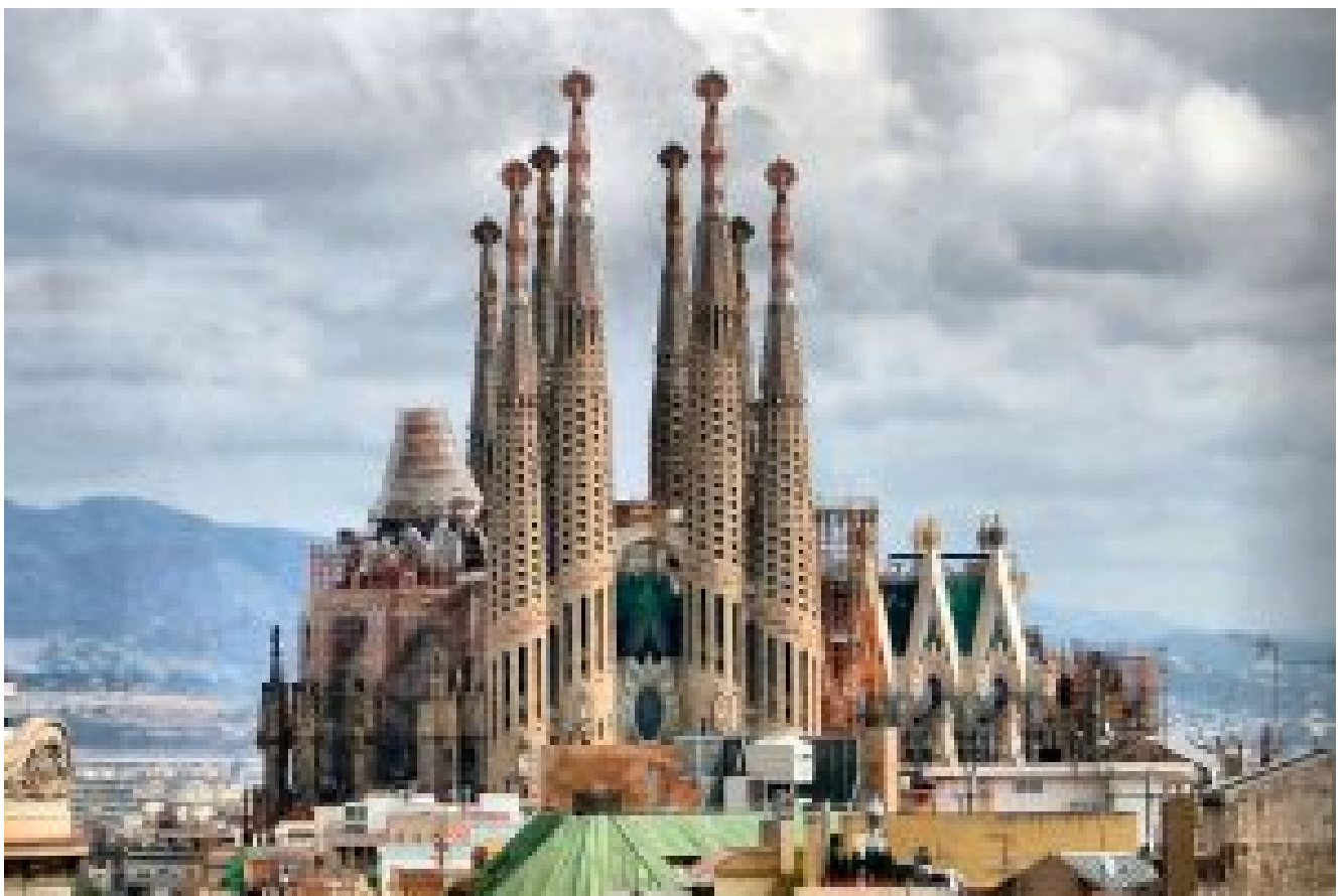
Construction fo the Sagrada Familia
