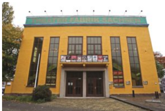
Exterior of the Theater- Fabrik-Sachsen
