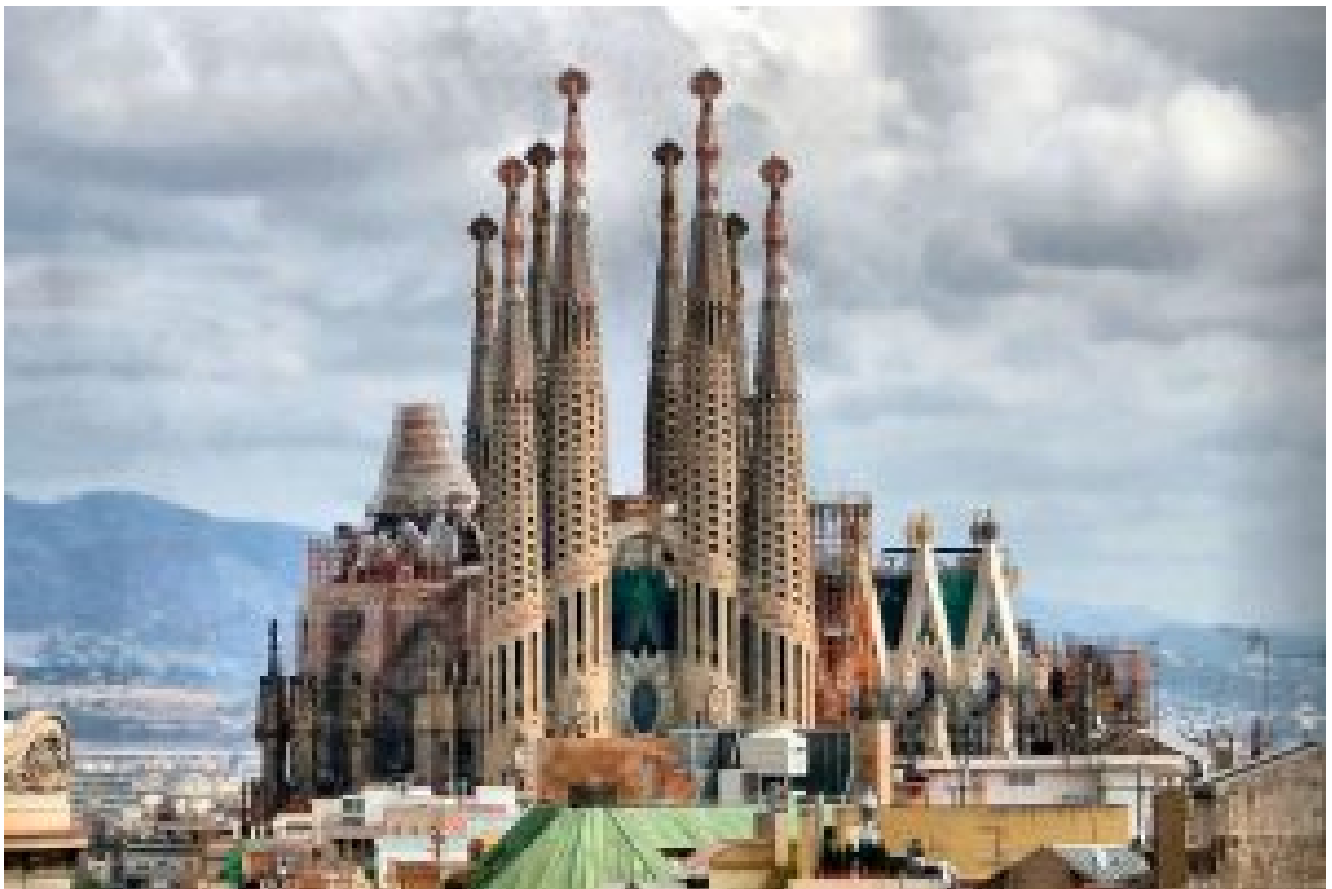
Construction fo the Sagrada Familia
