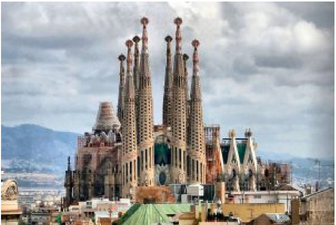
Construction fo the Sagrada Familia
