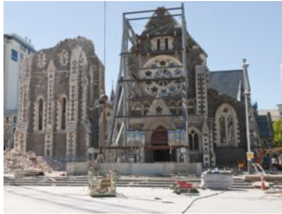
Cathedral west end bracing
