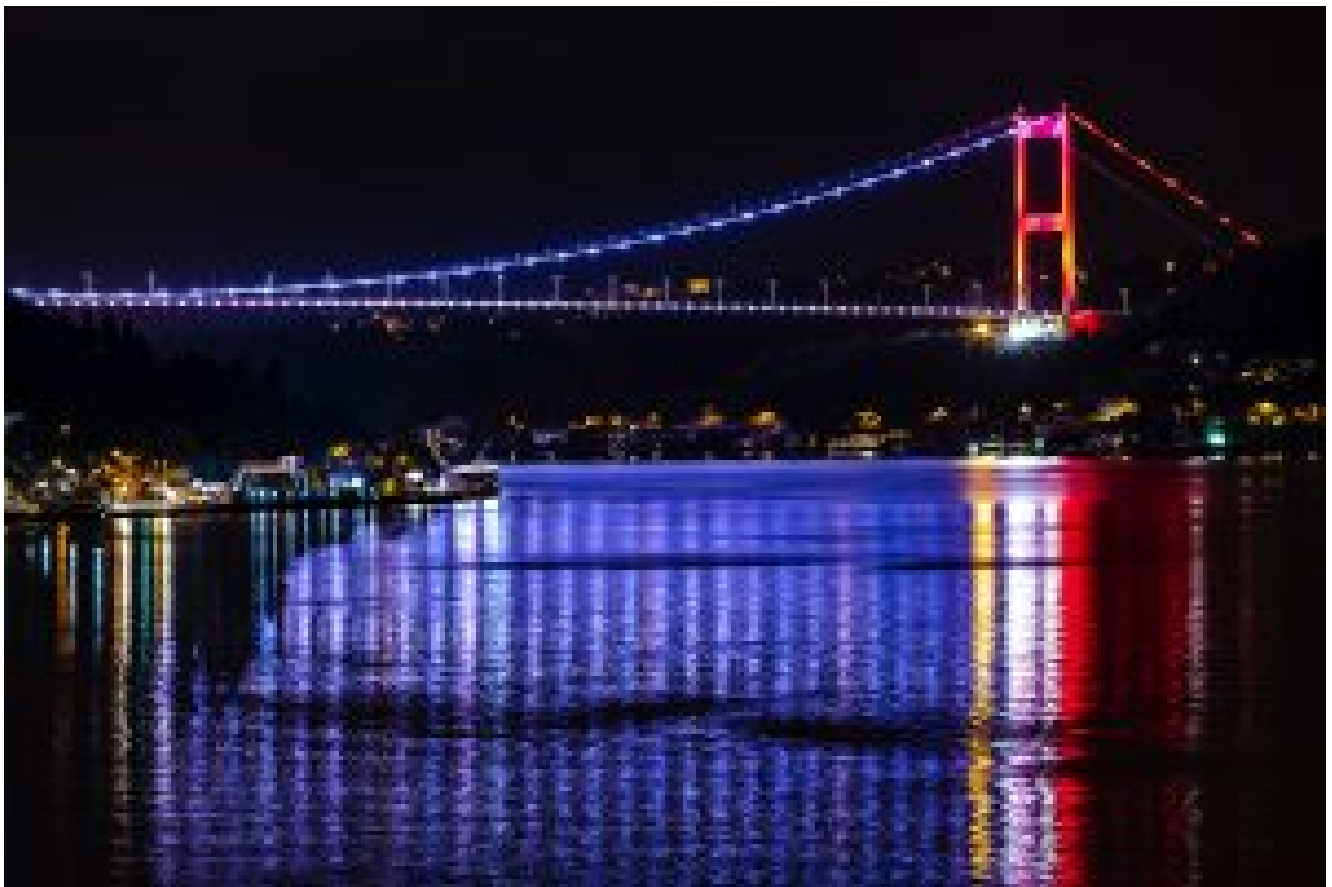
Bridge © Hulki Okan Tabak
