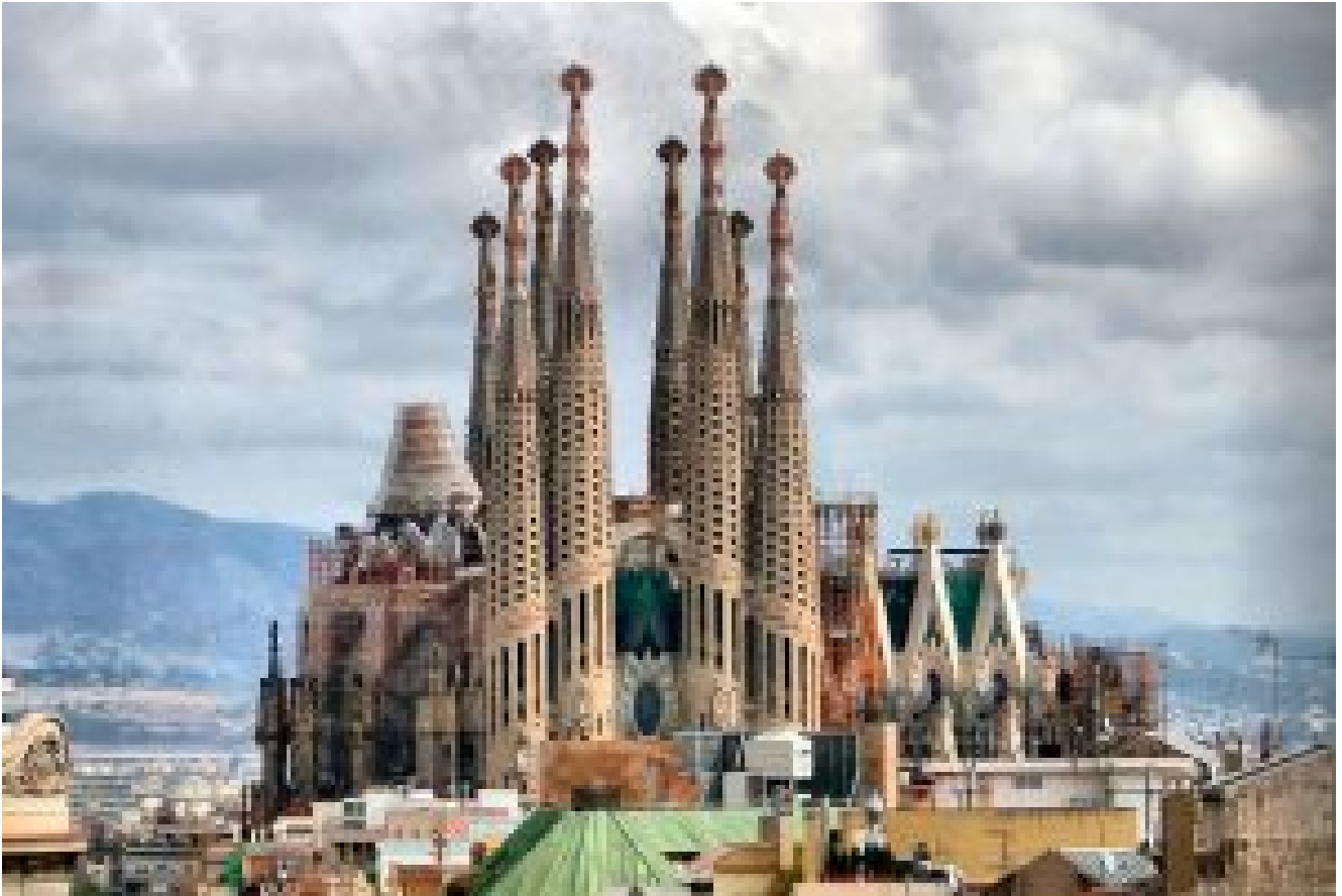
Construction fo the Sagrada Familia
