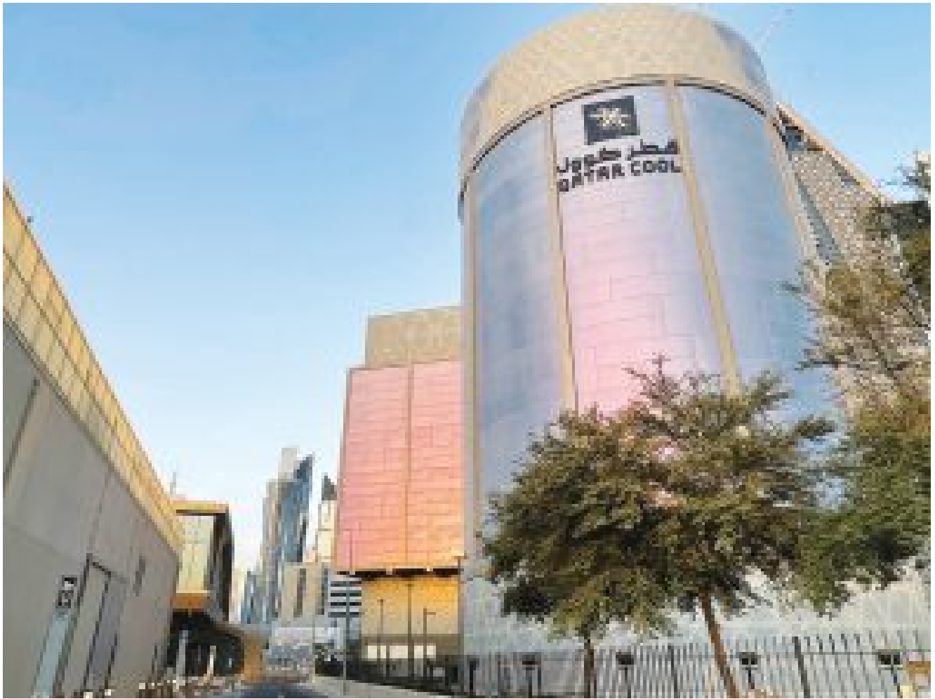
Qatar district cooling © Susie Billings
